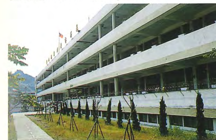
建德國小 Chan-Teh Primary School
